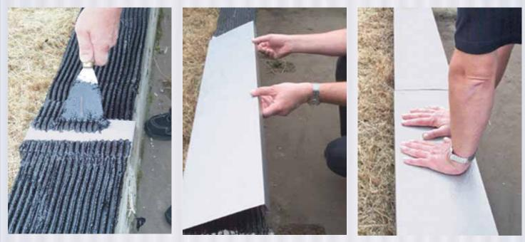
Adhesive bonding is practical solution in building applications, when stainless steel has to be fastened to masonry or natural stone.
